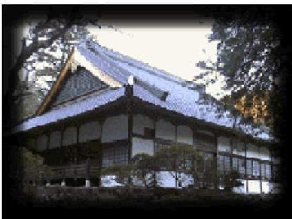
The Main Hall of Hosenji Temple was designated an Important Cultural Asset by the city of Kiryu on March 12, 2002. This one-storey building was constructed before 1726 in the “*irimoya*” or gabled style with copper roofing and has an area of 330 square meters.
