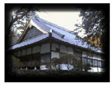
The Main Hall of Hosenji Temple was designated an Important Cultural Asset by the city of Kiryu on March 12, 2002. This one-storey building was constructed before 1726 in the "*irimoya*" or gablet style with copper roofing and has an area of 330 square meters.
